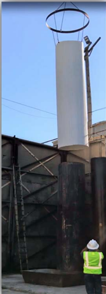
60"x20' Danby PL3F PVC liner Over PCCP pipe form
