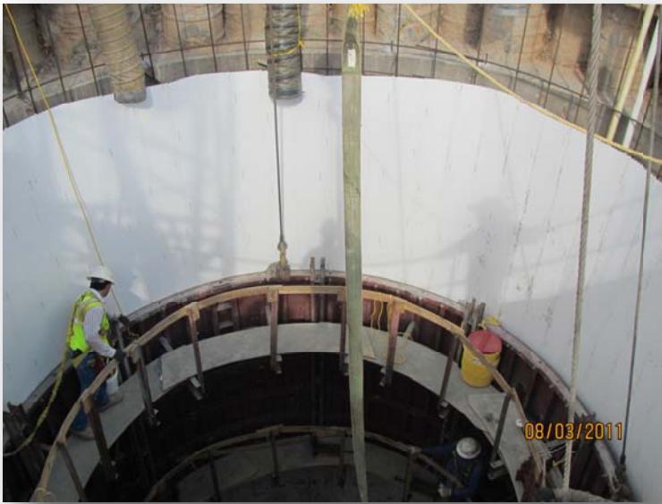
20' Dia. Structural Concrete Bypass Chamber lined using Danby PL3E PVC liner
