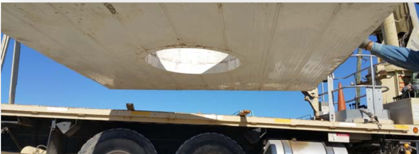
8' x 8' Concrete Lid HS20 load rated manhole lid lined with Danby PL3E PVC liner
