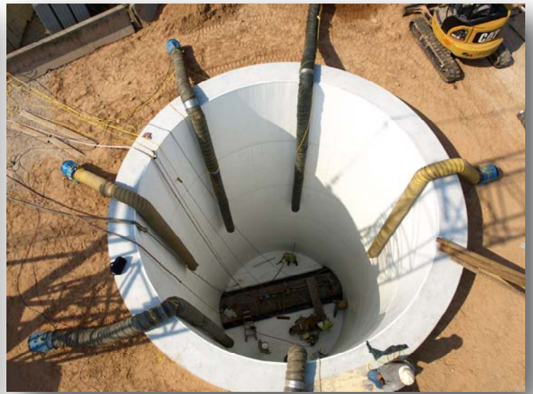
20' Dia. Structural Concrete Bypass Chamber lined using Danby PL3E PVC liner
