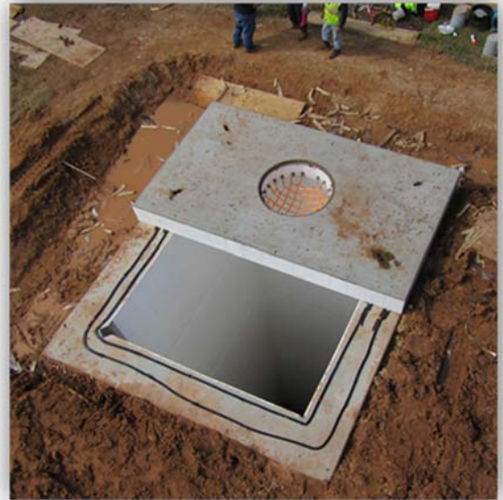
10'x16' Precast Concrete Structure Lid using Danby PL3E PVC liner (2 lids sections)
