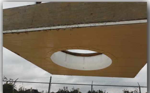
5x5 Manhole Lid lined with Danby PL3E PVC lining
