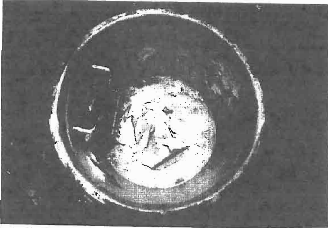
Figure 7. Epoxy coating failure.
